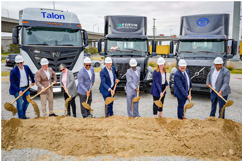
Image of the groundbreaking for Forum Mobility's charging depot from the Port of Long Beach press release.
